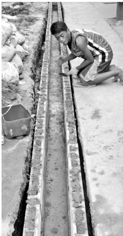
Implementation of canal lining in Barangay Ligdong III.
